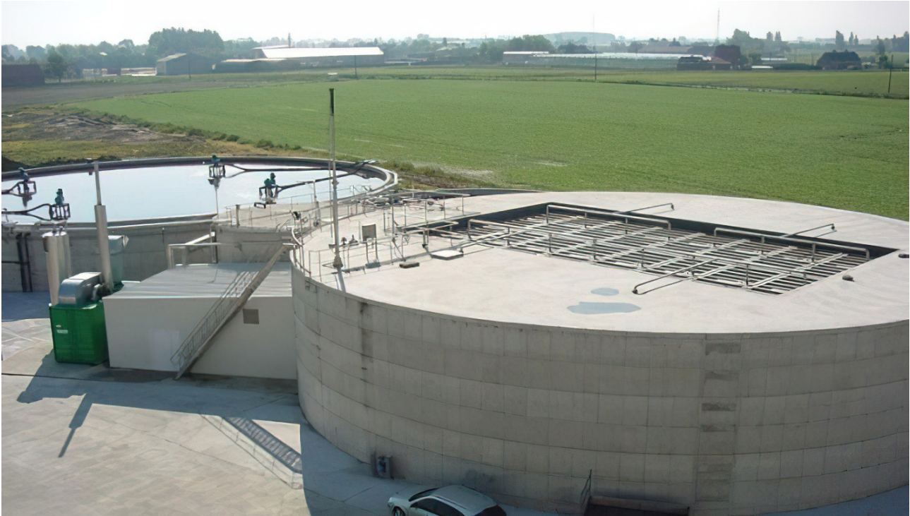
Figura 22. Reactor tipo UASB (Up-flow Anaerobic Sludge Blanket).
